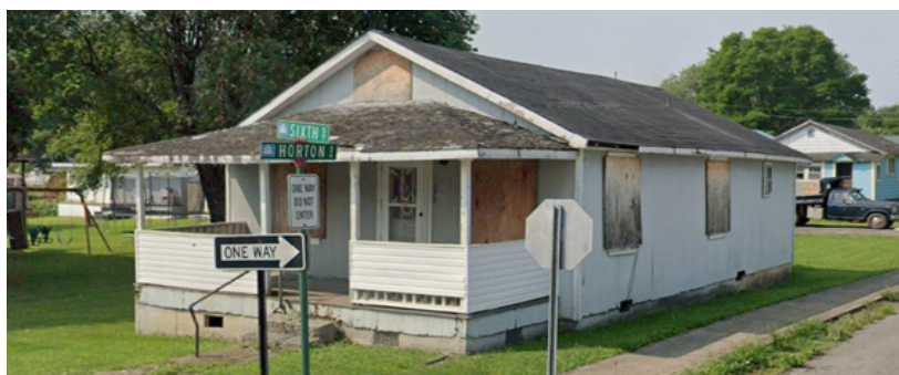
Figure 11: Example of low valued (Red Tag) structures in Floodplain of Rainelle
