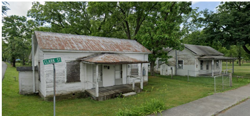
Figure 10: Examples of low valued (Red Tag) structures in Floodplain of White Sulphur Springs
